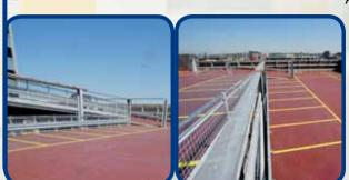
An alternative solution with a very tough, epoxy resin based, deck coating system, was recommended by NCC for use on the lower decks and ramps, because of the extremely high abrasion and wear resistance required.
